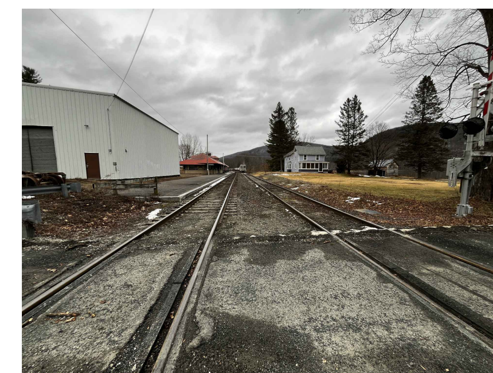
APPROXIMATELY 0.50 MILES OF RAILROAD SIDING ADJACENT TO THE BERKSHIRE SCENIC RAILWAY MUSEUM IN LENOX NEAR REACH 6
