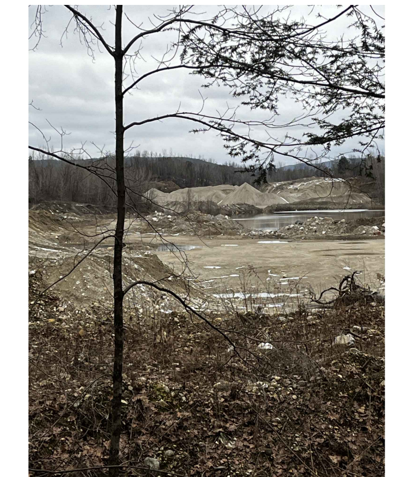
VIEW LOOKING TO THE SOUTHWEST OF THE UPLAND DISPOSAL FACILITY ALONG REACH 7A
