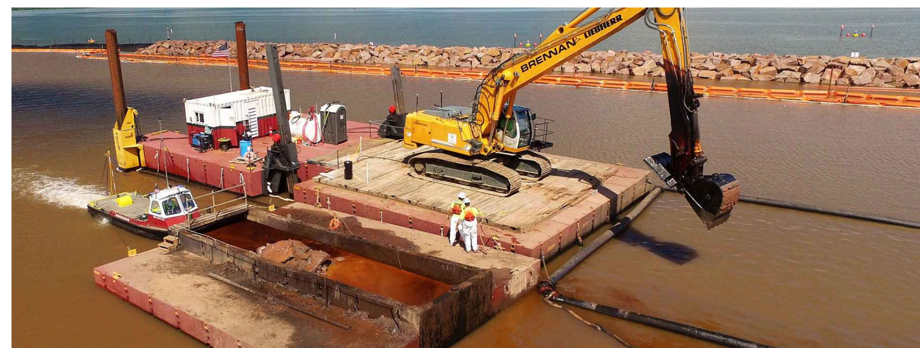
BARGE DREDGER WITH EXCAVATOR
